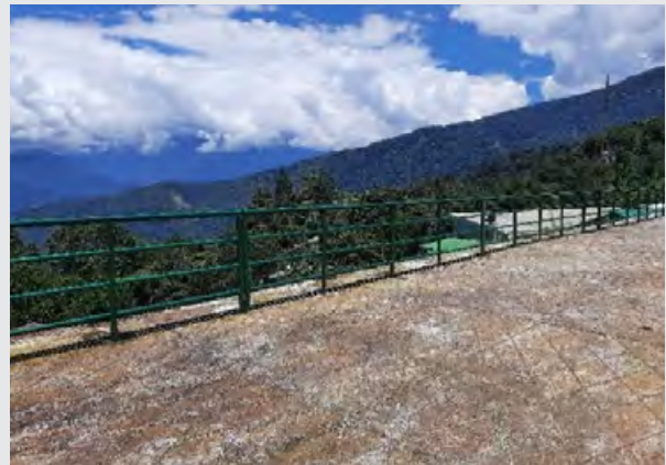
(b) Railing in front of Shed-I
