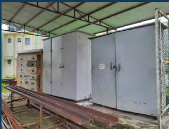
Fig 3. Installation of Electric Panel
